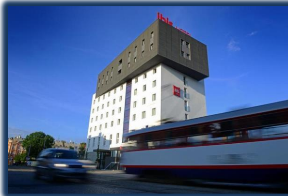
Figure 8: We stayed in a hotel in the city centre
